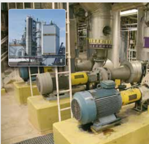
Easy-Laser® is used to align pumps and motors for all types of industries and installations. Correctly set-up and aligned machines are a requirement for achieving optimum service life and minimal energy consumption.
